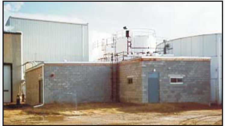
High-Rate Anaerobic-Aerobic SBR Plant
