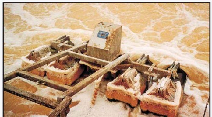
The AquaTec Decanter During Sub-Freezing Winter Operation
