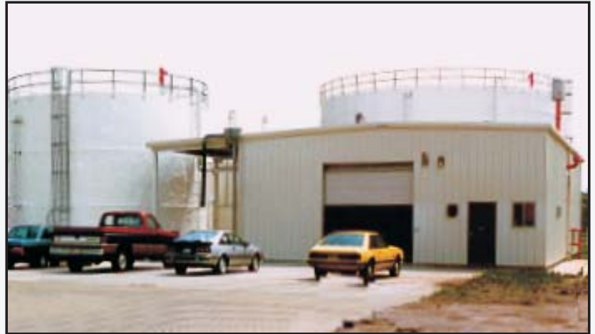
High-Rate Fixed-Film Anaerobic-Aerobic Plant
