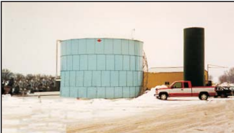
Single Tank SBR High-Rate Plant
