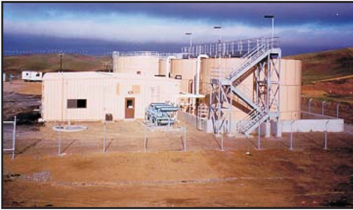
Multi-Stage Dual Reactor SBR Plant
